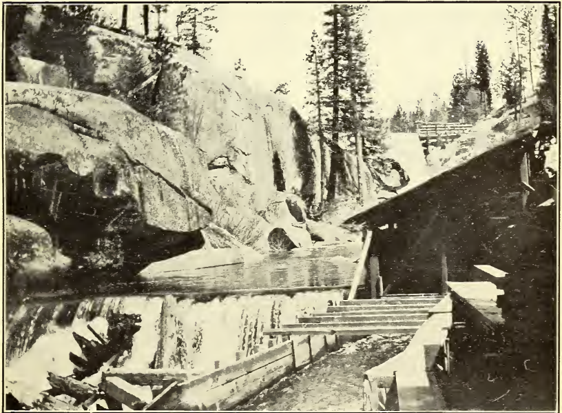
FIG. 2.—DIVERSION DAM AND FLUME BELOW LYONS DAM, SHOWING MAIN DAM IN DISTANCE.
